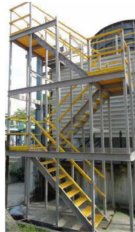
Platform with Handrails
